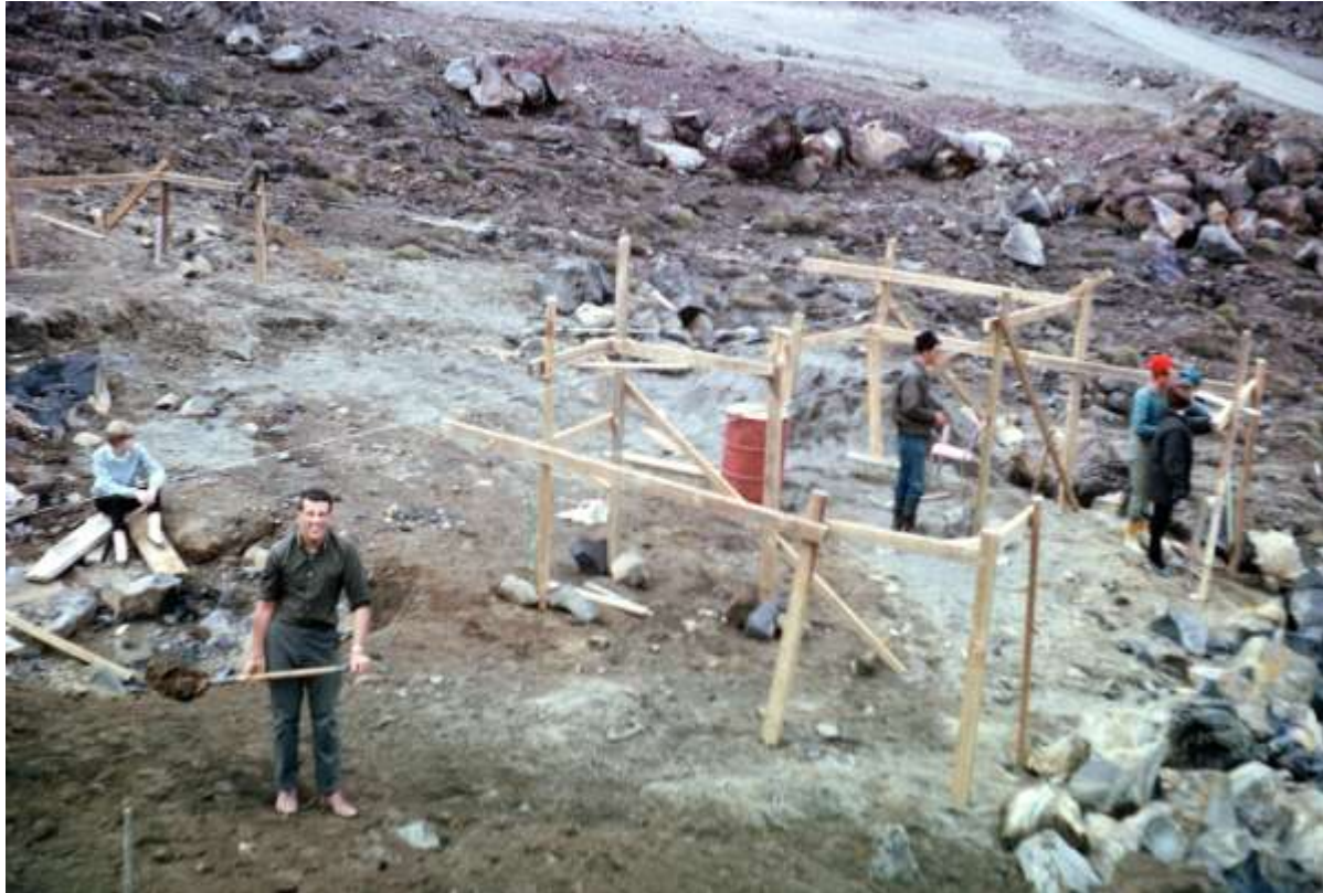
Figure 1 Profiles set, excavation is under way. 27 Feb 1965
